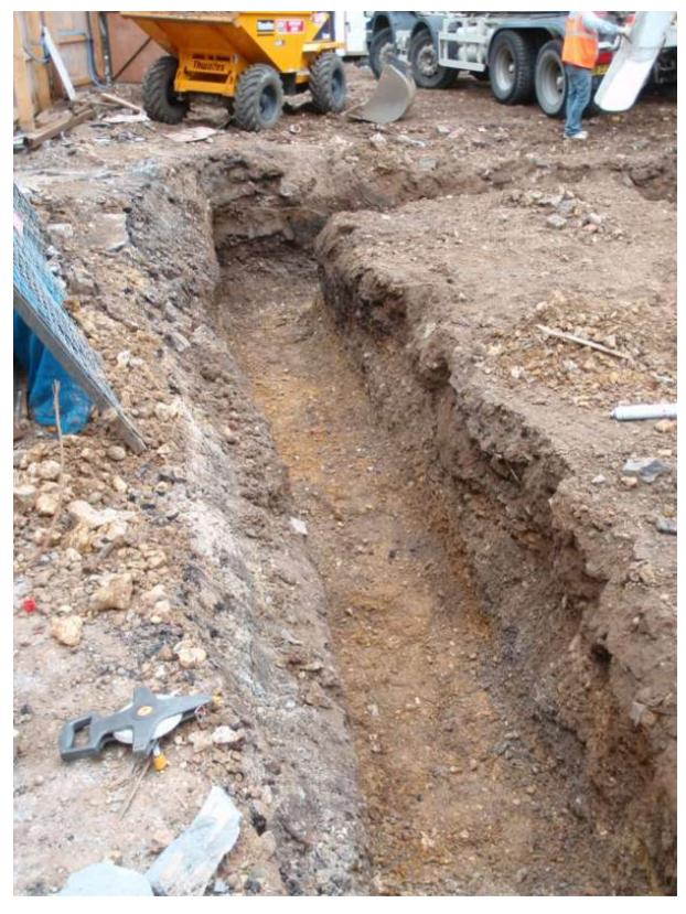
Plate 3. The site showing ground works (foundation trenches) facing east
